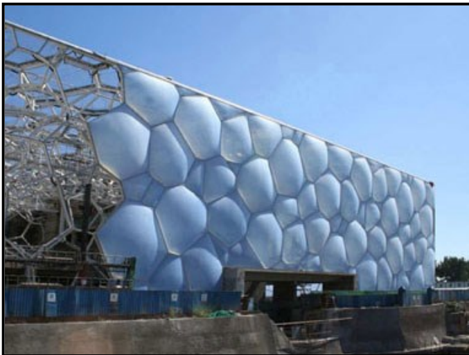
FIGURE 8a: Chris Bosse (PTW Architects), Watercube , Beijing's National Swimming Centre, 2008.
