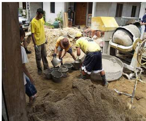
Mixing cement using a mixer.
