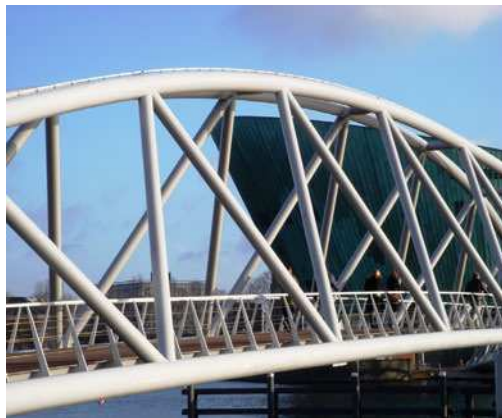
A bridge made of metal.
