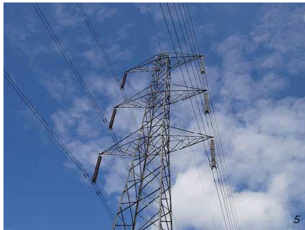
A pylon is a frame structure that supports electricity lines.
