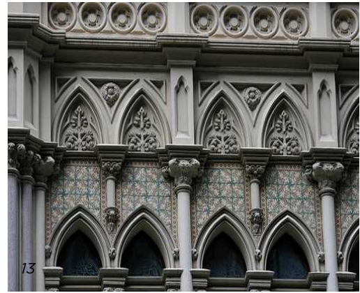
Decorative carvings and columns made from sandstone on the front of a building.
